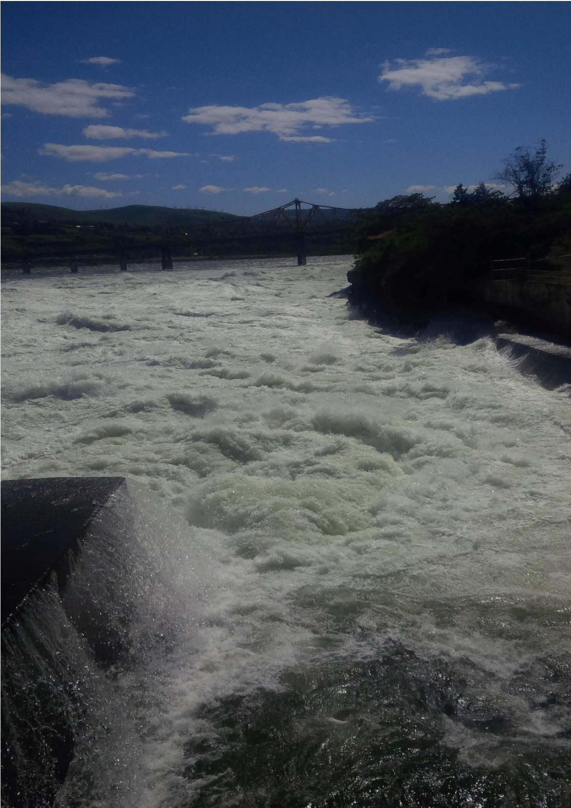
High spill turbulence continues at north entrance
